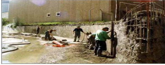
Drainage channel repair with shotcrete fibre reinforced located in Bankstown, Australia. (Source: Novocon, 2000)
