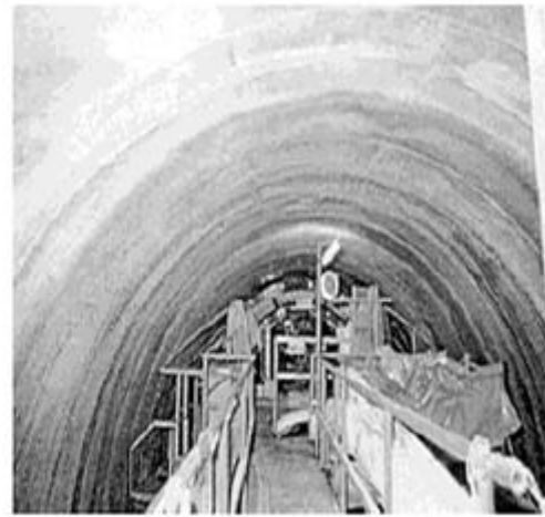
ECL in Ojiya Headrace tunnel. 13
